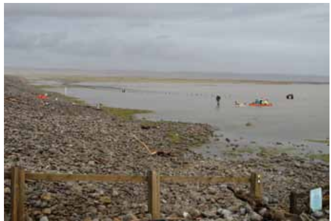
A breach at the southern end of the pebble ridge after winter storms (January 2014) Pebbles have filled the play area with its pirate ship (left) and sea water has flooded the flat land behind the ridge (right) © Tara Sanders
