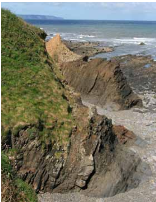
Upended rocks visible on the cliff edge Dave Edgcombe © North Devon AONB
