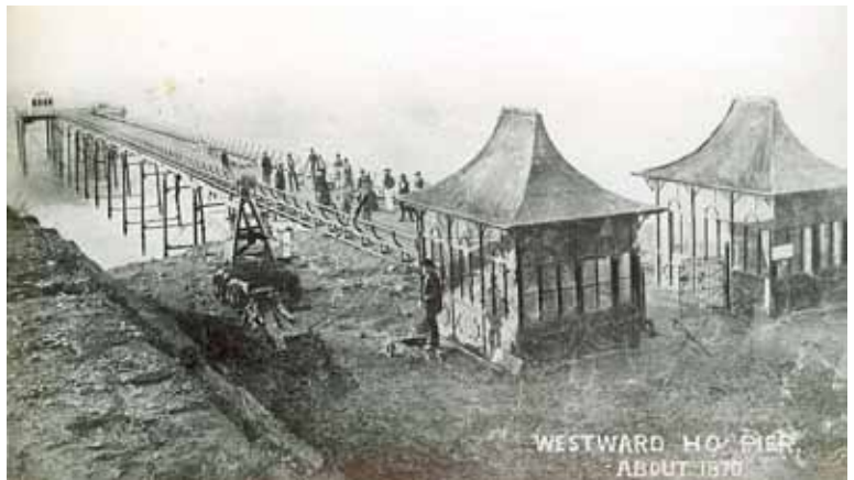
Westward Ho! pier under construction (1870) Courtesy of Westward Ho! History Group
