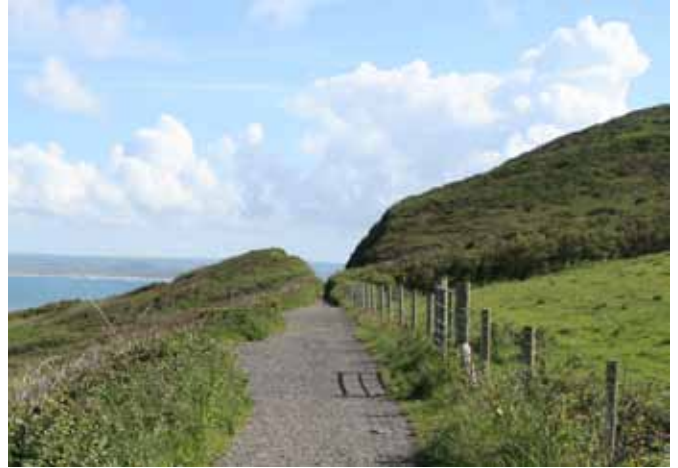
Old railway line and cutting Dave Edgcombe © North Devon AONB
