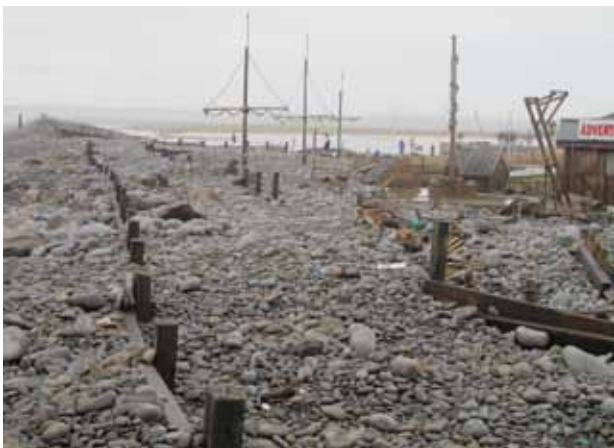
A breach at the southern end of the pebble ridge after winter storms (January 2014) Pebbles have filled the play area with its pirate ship (left) and sea water has flooded the flat land behind the ridge (right) © Tara Sanders
