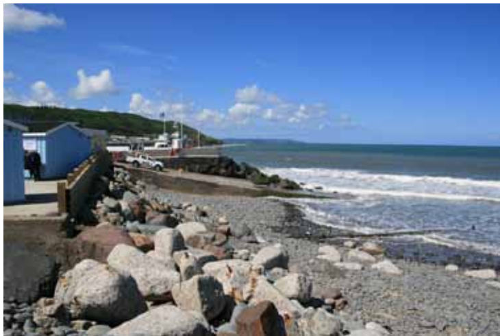
Large boulders protect the concrete seawall Dave Edcombe © North Devon AONB
